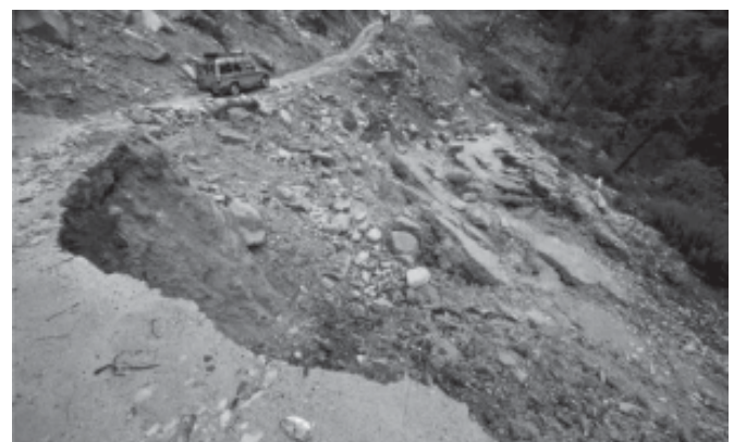
Fig.3. Landslide Due to Heavy Rains
